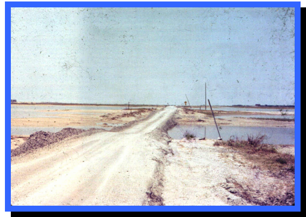
HIGHWAY 361 AFTER EMERGENCY REPAIR Temporary repairs after Celia.
