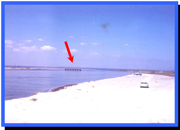
HIGHWAY 361 BRIDGE AFTER BEULAH Note the bridge isolated in the channel.
